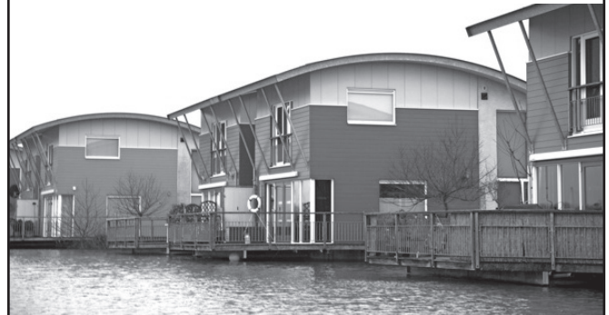
How the Dutch do it ... “Amphibious” houses at Maasbommel, on the River Meuse, which rise on the flood, up to 5.5 metres if necessary, float and then subside - no effort required.
